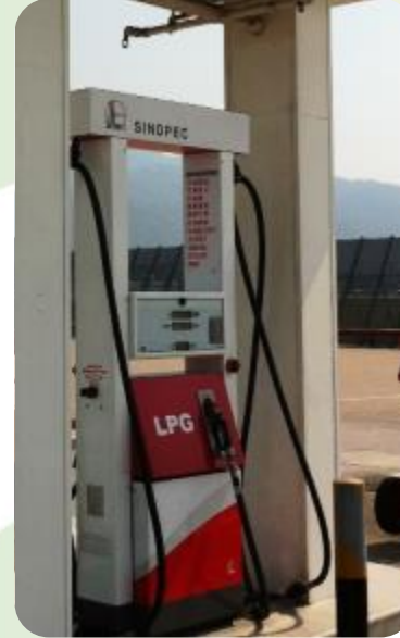
LPG refueling station
