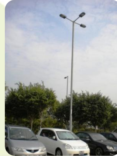
Solar Panel Trial (car park 2)
