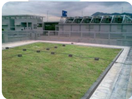
Green roof at seawater pump house
