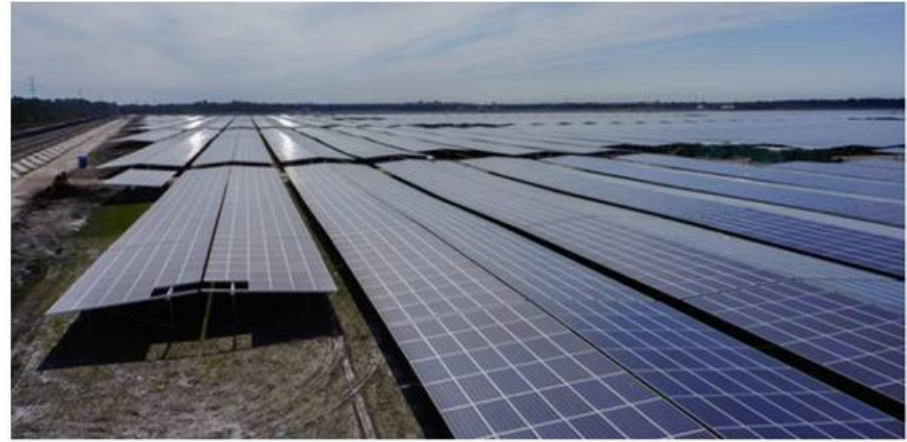
Image: Neoen (300MW project in Cestas, France, developed by Neoen with east-west orientation for maximum land efficiency)
