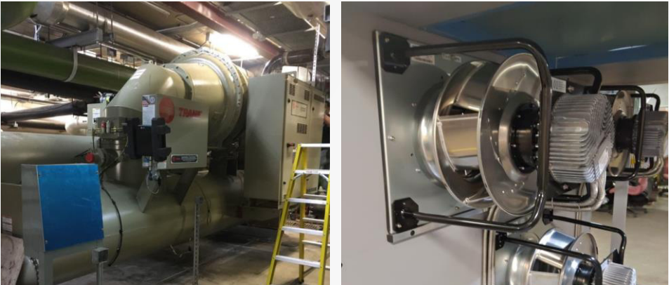
Equipment Replacement & Upgrading e.g. EC Motor Plug Fans – estimated >7.5M kWh savings
