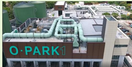
DELIVERY OF ORGANIC FOOD WASTE TO OPARK.1 FOR ELECTRICITY GENERATION
