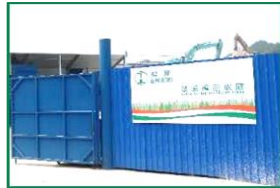
Glass Recycling Plant (Tuen Mun)
