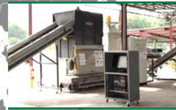
Waste Sorting & Recycling Centre (Fanling)
